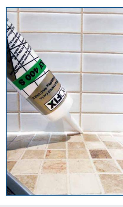
Buildings are under continuous stress, which affects their structure, and can cause cracks in the grout lines at wall junctions, between walls and floors, between counters and walls, etc. Although in most cases the consequences are purely aesthetic, the appearance of cracks in showers, bath surrounds, and kitchen counters can be more problematic. PROFIX offers two types of products to counter this phenomenon: POLY 400 S and POLY 400 U.
